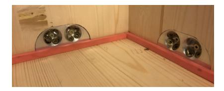
Fixing with SHERPA CLT connector
